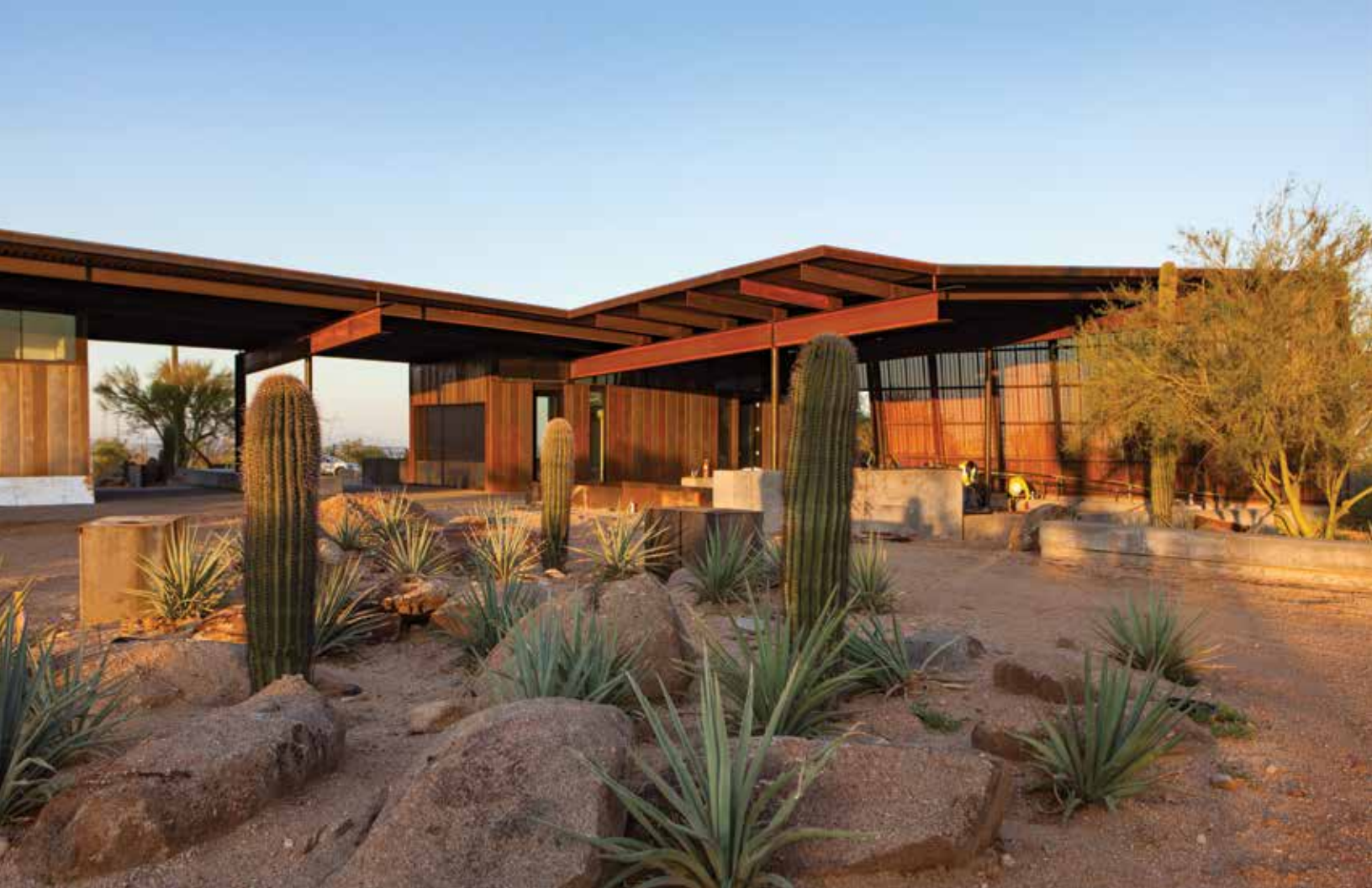
Construction of the Pima Dynamite Trailhead began in August 2020 and will be completed in September 2021. Photo by Dennis Eckel
