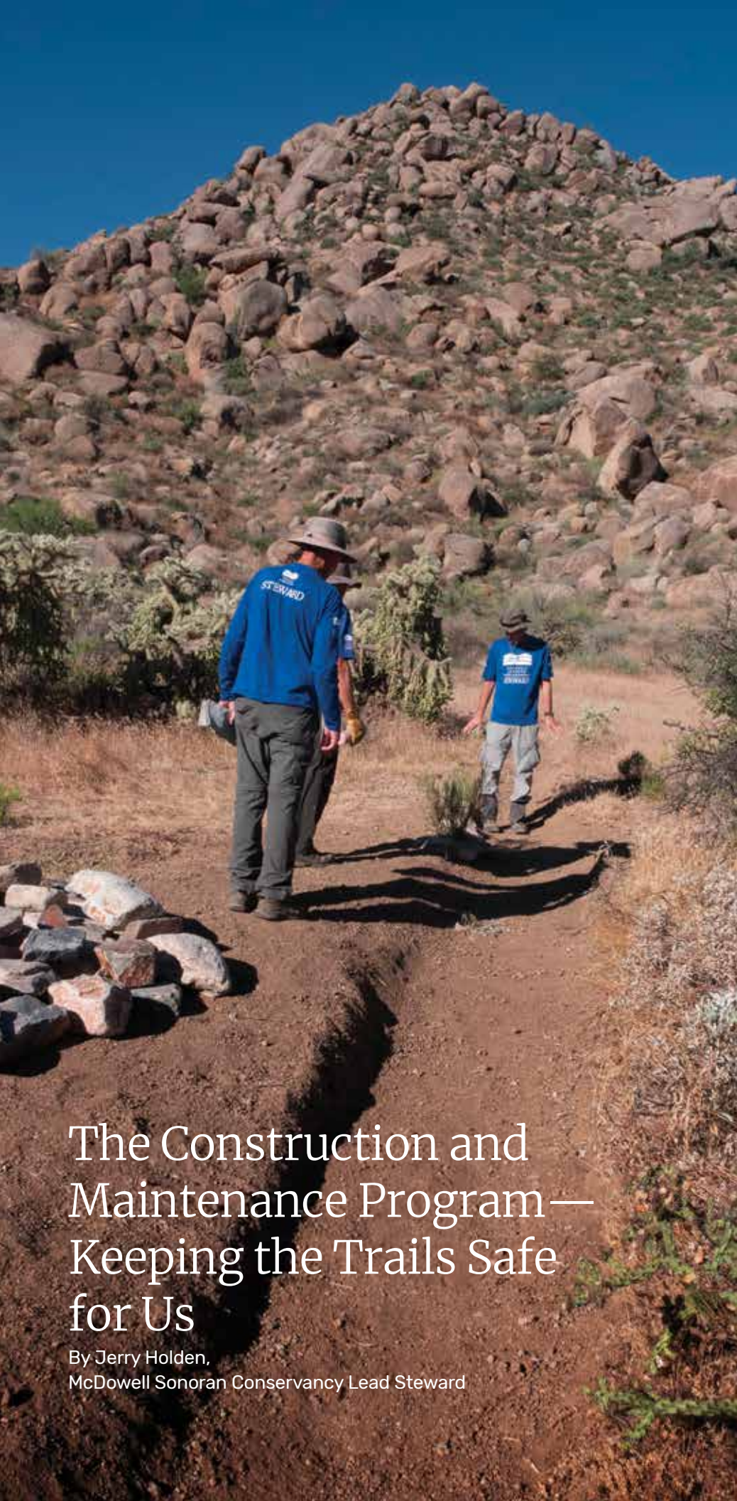
Drainage corridors are used to divert water across the trail. This Construction & Maintenance (C&M) crew will armor this drainage corridor on Marcus Landslide Trail with the rocks shown in the photograph. Photo by Lynne Janney Russell
